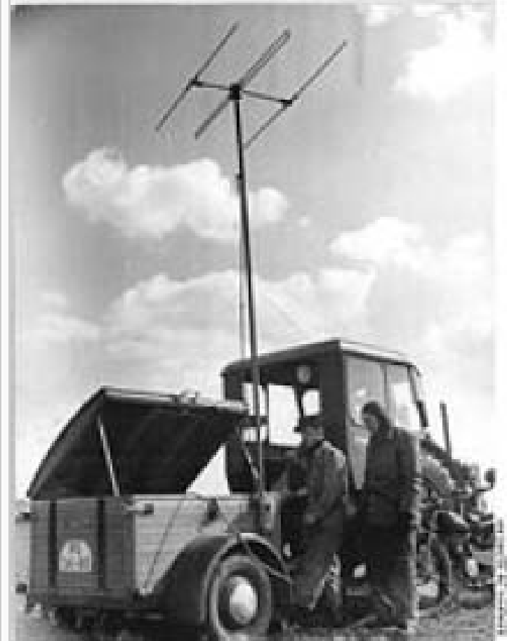
Yagi antenna used for mobile military communications station, Dresden, Germany, 1955
